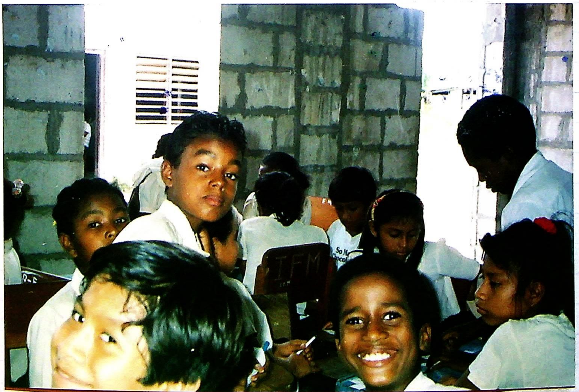
Classroom realities, Unfinished walls and windows.
